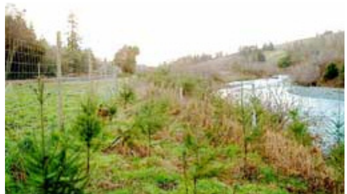
FL-04, 01/28/02, STA 5.75-7.16, view similar to above
